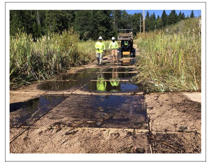
**Photo 2**: Mats were installed along the north end of the transmission line alignment in accordance with APM-BIO-5.
