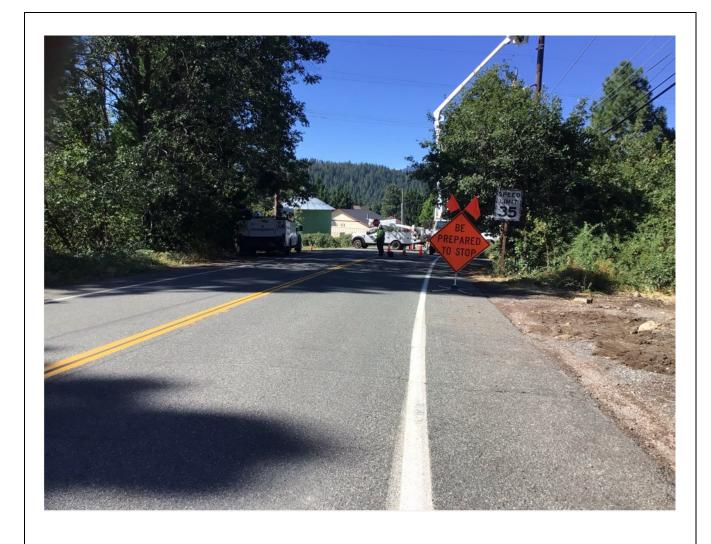
**Photo 5:** Traffic controls were observed in place on W. Ream Road for transmission pole 2/48 installation per APM TT-1.
