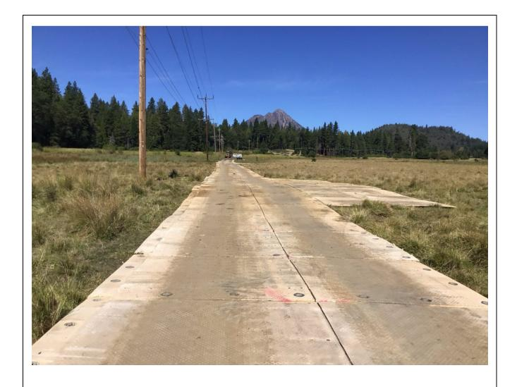
Photo 3: Mats were installed along Hatchery Road in accordance with APM-BIO-5.
